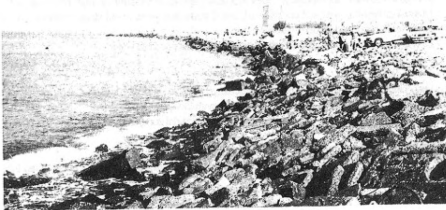
Fig. 13. Photograph of shoreline type 6, riprap (boulder) structures.
